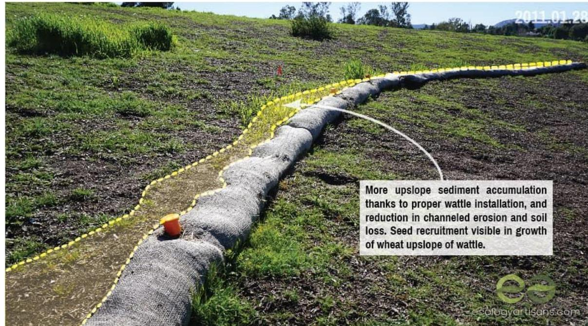
More upslope sediment accumulation thanks to proper wattle installation, and reduction in channeled erosion and soil loss. Seed recruitment visible in growth of wheat upslope of wattle.
